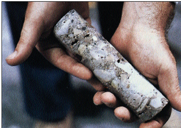
Figure 2. Drilled cores give information about floor thickness, height of wire mesh, and location of delaminations.
