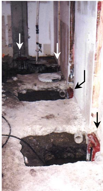
These photographs show the Atlas 2-Piece Resistance Piers installed along internal basement walls. Each pier was driven to a suitable bearing stratum below the poor soil. After reaching refusal, each pier was individually tested to a load
