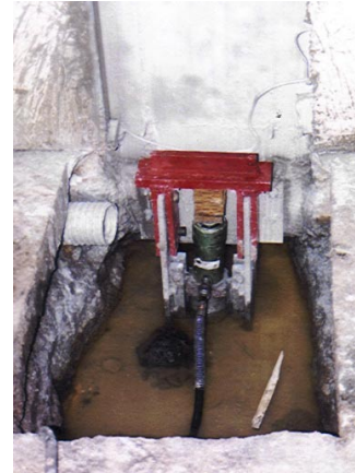
These photographs show the Atlas 2-Piece Resistance Piers installed along internal basement walls. Each pier was driven to a suitable bearing stratum below the poor soil. After reaching refusal, each pier was individually tested to a load
